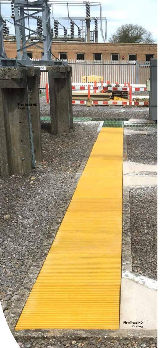
LK Flowtread HD series pultruded open mesh grating has been engineered to carry vehicular loads.
